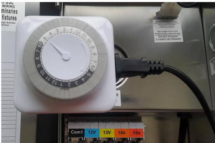
Insert the timer into the outlet on the transformer as shown.
